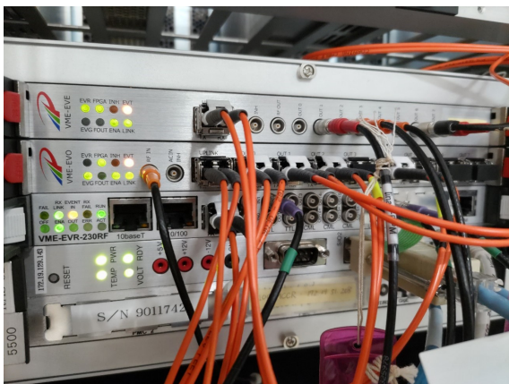
Figure 4: Picture of MR sub-timing station.
