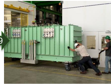
9 Transport into bunker
