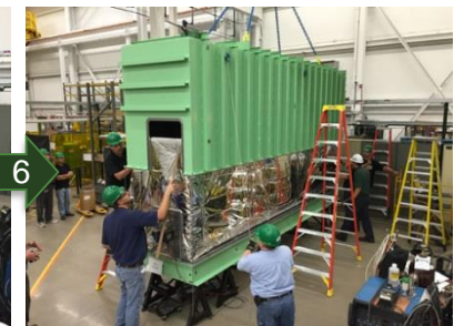
6 Vessel cover installation
