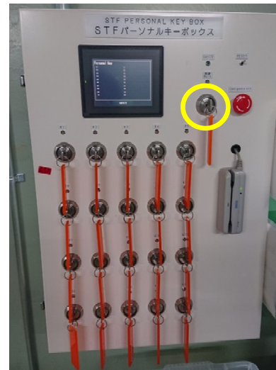
Figure 4: STF tunnel personal key box.
