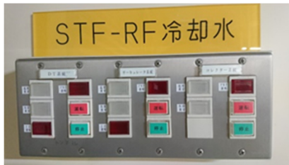
Figure 2: Cooling water operation switch.
