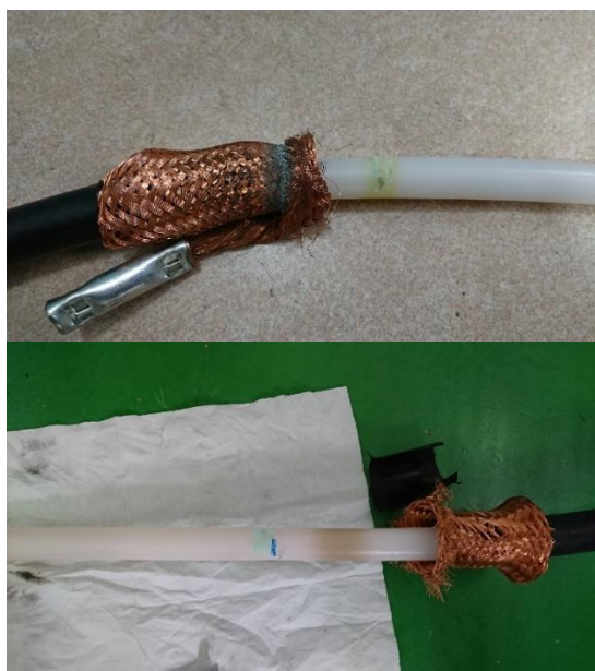
Figure 1: High-voltage cable with insulation failure. Top and bottom pictures are terminals in HVS and klystron sides, respectively.
