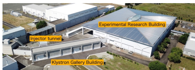
Figure 1: NewSUBARU synchrotron light facility.
