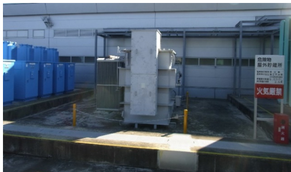
Figure 9: Storage location of the transformer-rectifier unit.
