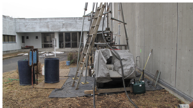
Figure 2: Preparation of boring devices and a boring point in the 17.6 m north from the entrance of the injector linac building.
