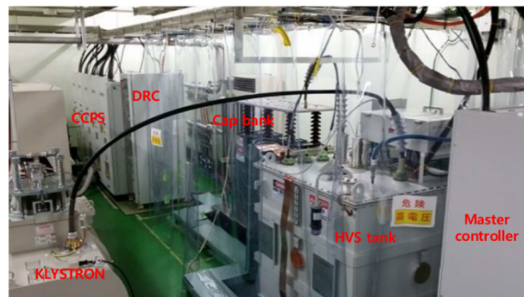
Figure 12: The modulator power supply in iBNCT.
