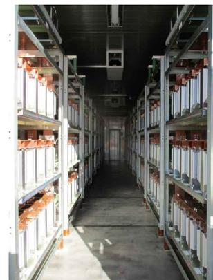
Figure 6: Metal racks installed in the marine container.
