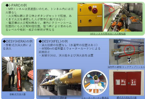
Figure 17: Fire protection in J-PARC and DESY.
