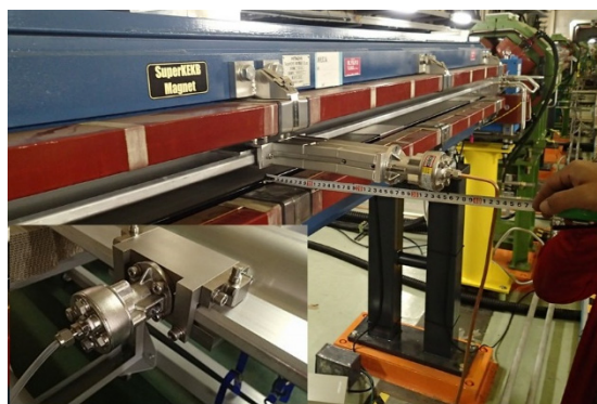
Figure 8: Knocker attached to a beam pipe for bending magnet.
