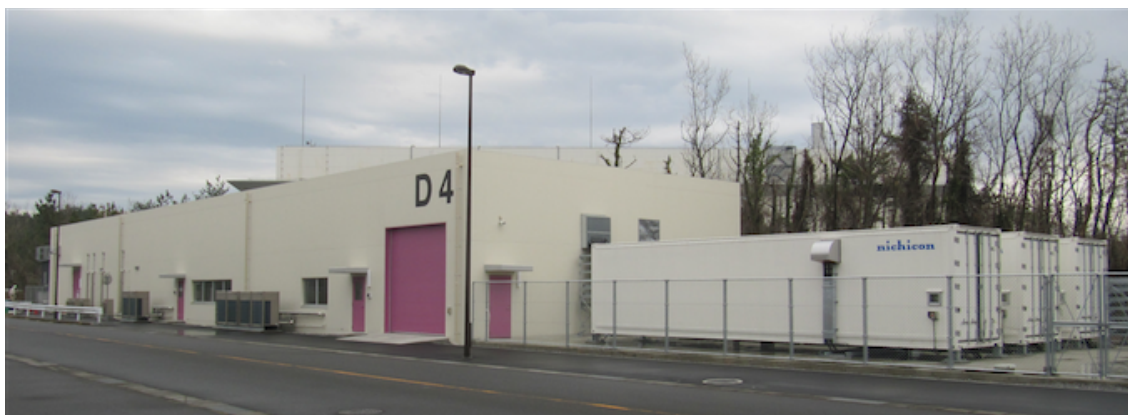
Figure 2: Picture of building which is installed power converters (left side) and containers for installing capacitor banks (right side).
