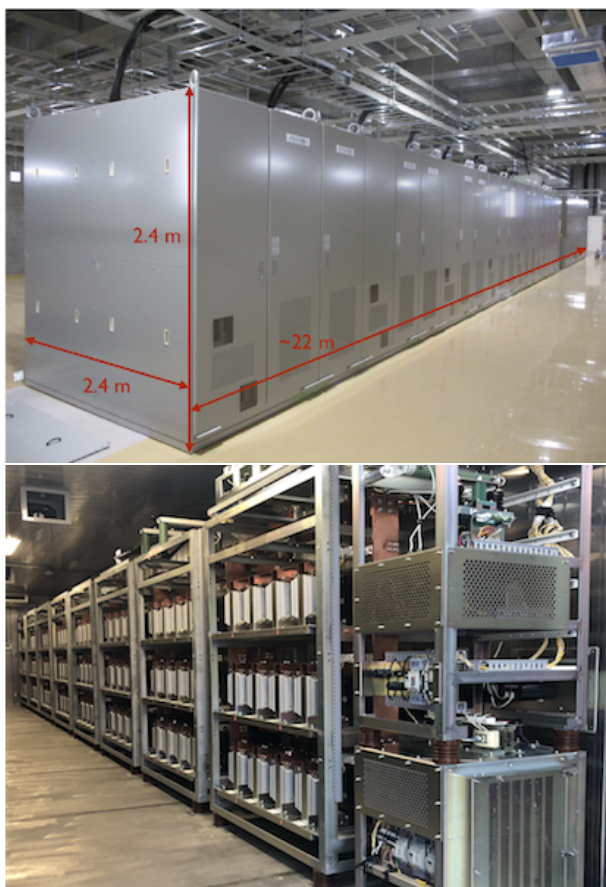
Figure 1: Pictures of power converters (upper) and a capacitor bank (bottom) installed in a container for the bending magnet family in J-PARC MR.
