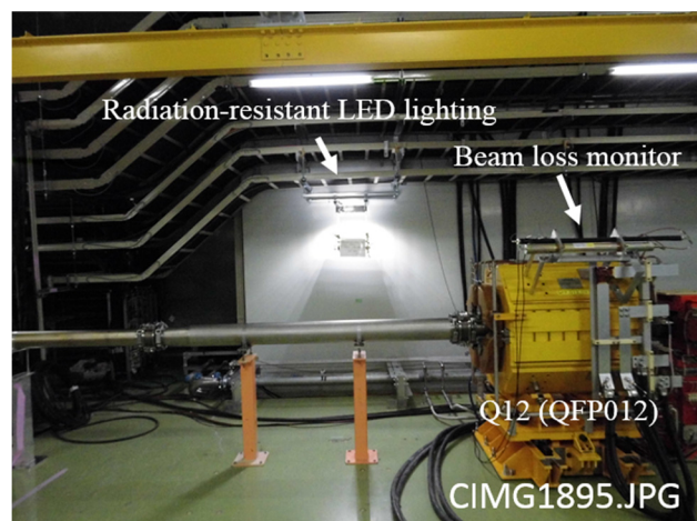
Figure 1: Setup of the Radiation-resistant LED lighting.
