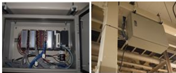
Figure 1: Picture of the data logger provided with the communication unit, power supply unit and input units.
