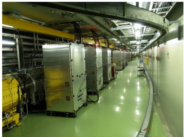
Figure 2: Nine sets of new FT3L magnetic alloy loaded cavities.
