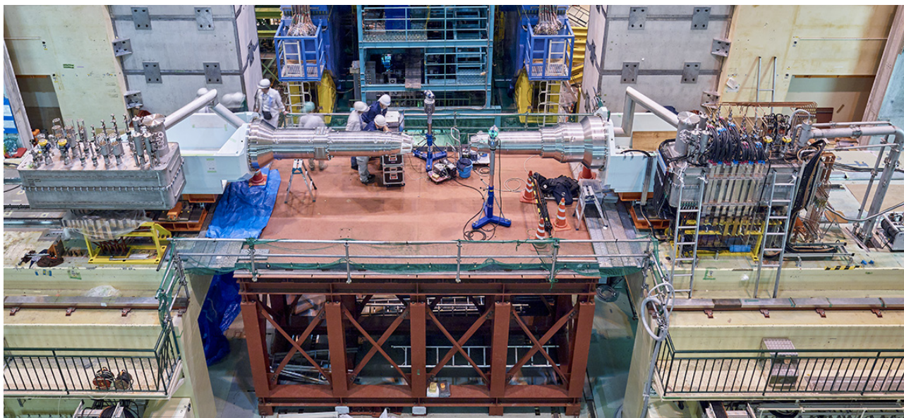
Figure 1: Overview of the final focusing superconducting quadrupole magnets after the installation in the IR region. The right-hand side magnet shows so called QCSL and the left-hand side magnet shows QCSR.
