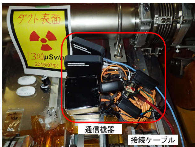
Photo 3: The equipment near the beam duct pipe (Test 1).
