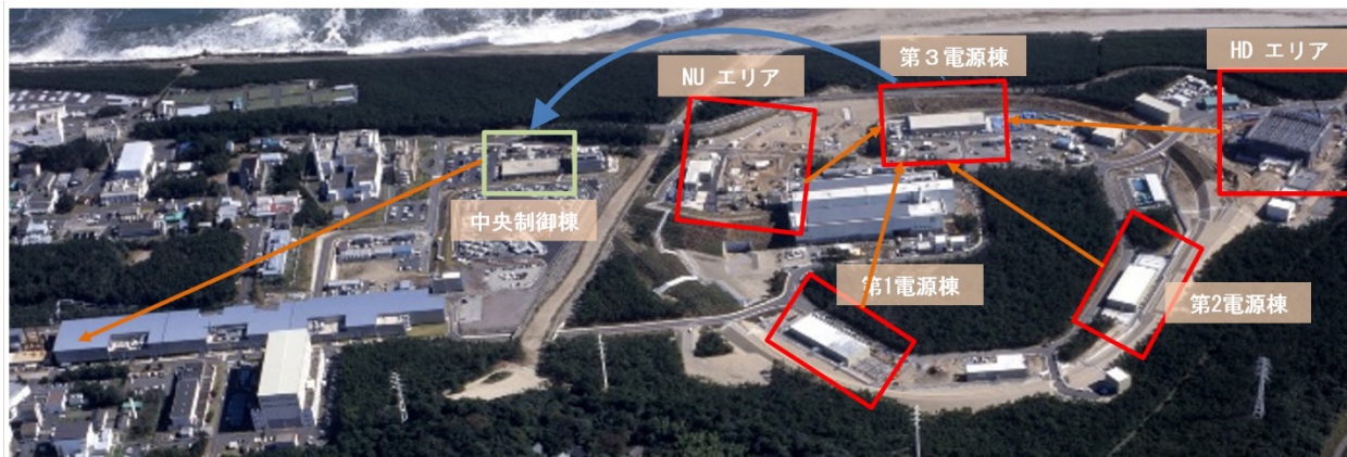
Figure 1: Red box shows the location where MPS equipment is.
