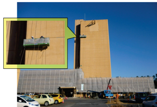
Figure 7: Repair work of the outer wall.
