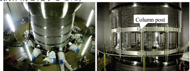
Figure 4: Exchanging work of insulating column posts.
