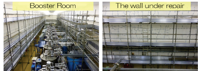
Figure 6: Repair work of the wall in a building.
