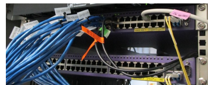
Figure 4: Edge switches.
