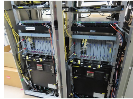
Figure 2: Core switches.
