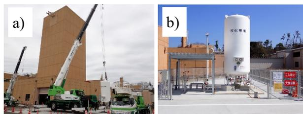
Figure 2: a) Photo of construction work of cold evaporator (CE) of liquid nitrogen. b) Completed CE.
