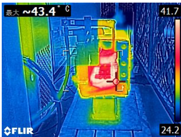
Figure 3: Heat distribution image by an infrared thermography camera.
