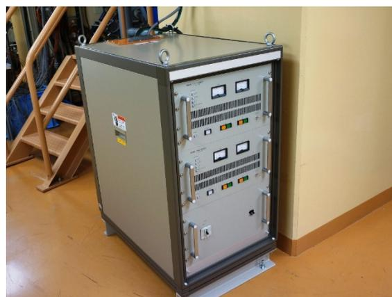
Figure 5: Picture of the newly installed 1 kW transistor amplifier for the cyclotron RF system.
