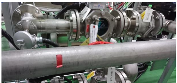
Figure 4: Enlarging RFQ cooling-water pipe diameter to increase flow rate, before (top) and after (bottom) the refurbishment.
