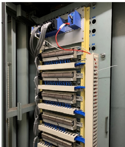
Figure 4: Relay system has been renovated with relay terminals. These are monitored and controlled by PLC.
