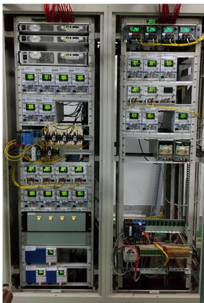
Figure 2: Photograph of new power supplies for magnets.
