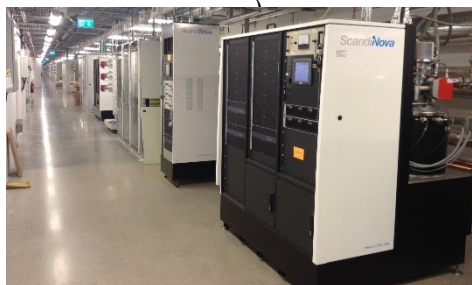
Figure 11: Klystron gallery with K300 modulator.
