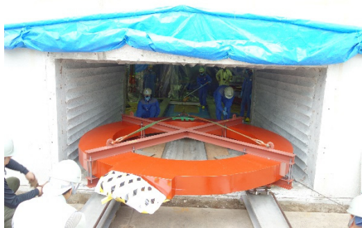
Figure 5: Carrying work of the new main coil.
