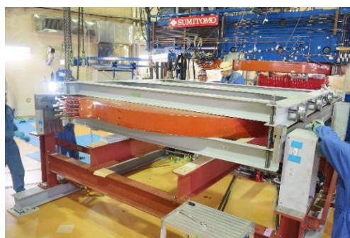
Figure 4: Removing the main coil of the cyclotron.
