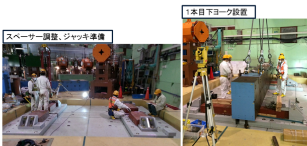
Figure 5: Alignment of the bottom yokes.
