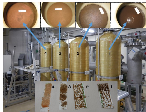
Figure 2: Contamination of RI4 water flow system.
