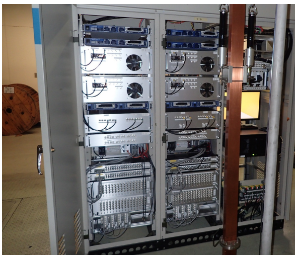
Figure 6: Photograph of the pulsed steering and quadrupole magnet power supply and control system. The control system is based on the PXI and CompactRIO buses. The control software comprises NI LabVIEW and EPICS frameworks.
