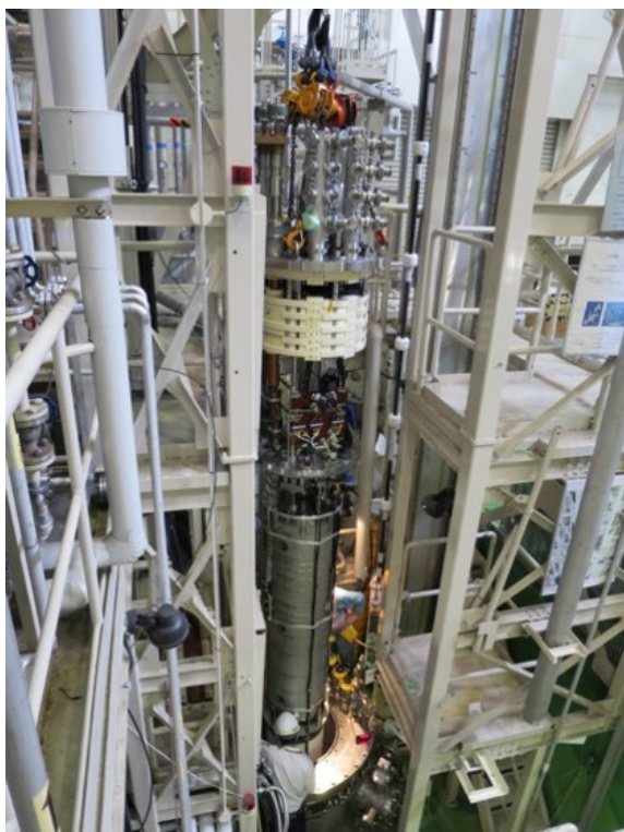
Figure 1: Insertion of the 2 m model magnet to the 9 m-deep-vertical cryostat.
