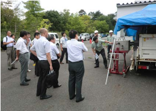
Figure 9: The photograph of the non-destructive testing for a 60-cm thickness concrete demonstrated in an open field.
